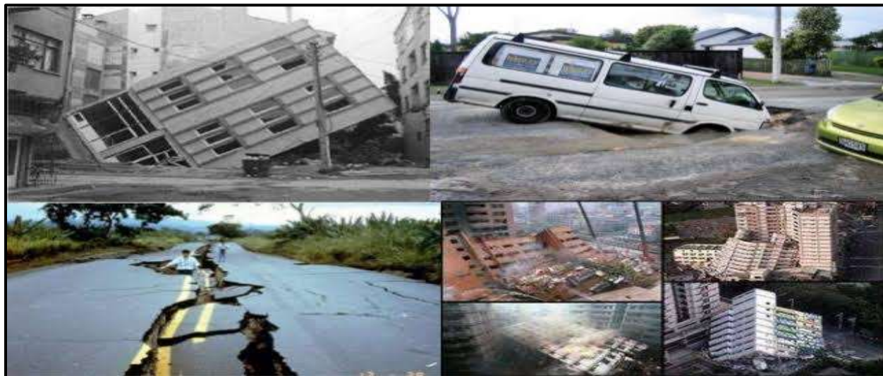
Fig. 5.1 Soil Liquefaction
